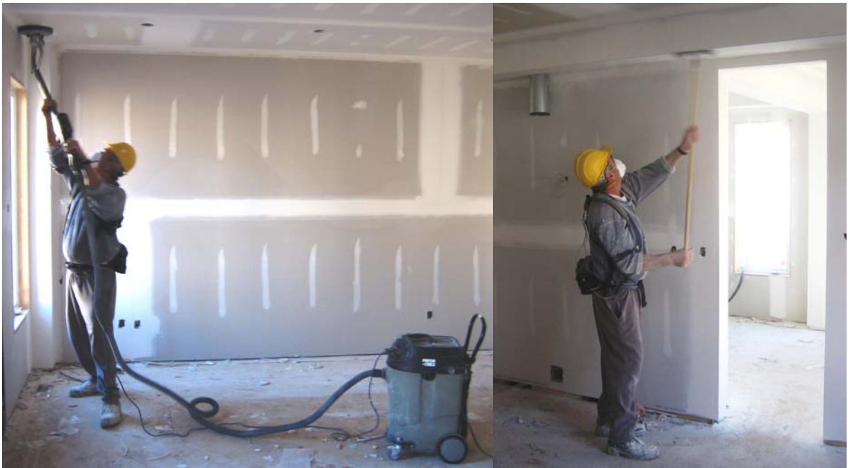
Figure 1: Sanding skimmed drywall using a mechanical sanding-vacuum machine (left), and a sanding pole (right).
